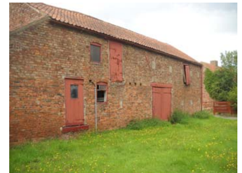
Plate 9 Barn at Manor Farm
